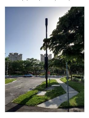
Additionally, the PWF will be consistent with Town Code with respect to height, with the facility heights limited to 35 feet within the Gulf of Mexico Drive ROW, and 25 feet within other Town ROW's. Spacing will also meet requirements of being no closer than 60 feet from adjacent lighting deployed by the Town or another freestanding personal wireless service pole (Note: Recently amended as part of Ordinance 2021-16.).
