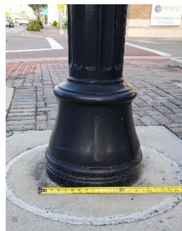
Manatee County Downtown Bradenton ~25-ft. poles with ~4-ft. arms Pole diameter of ~ 8 inches Base diameter 16 inches
