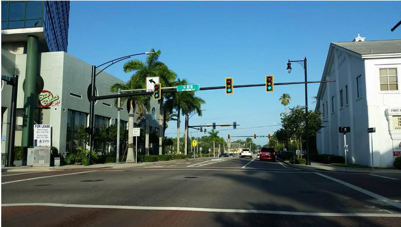
Downtown Bradenton ~ 25-ft. poles with ~15-ft. arms ~ fixture mounted to Mast Arm Base
