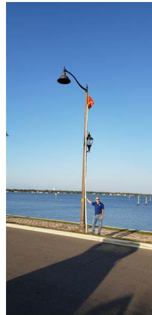
Manatee County Green Bridge ~25-ft. poles with ~8-ft. arms Pole diameter of ~ 8-9 inches Concrete Base diameter ~18 inches
